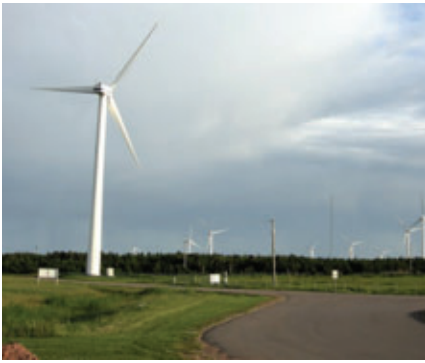
Canadian Wind Energy Institute, North Cape, P.E.I.
